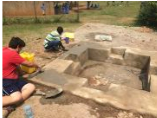
Oliver working on the guesthouse fire pit
