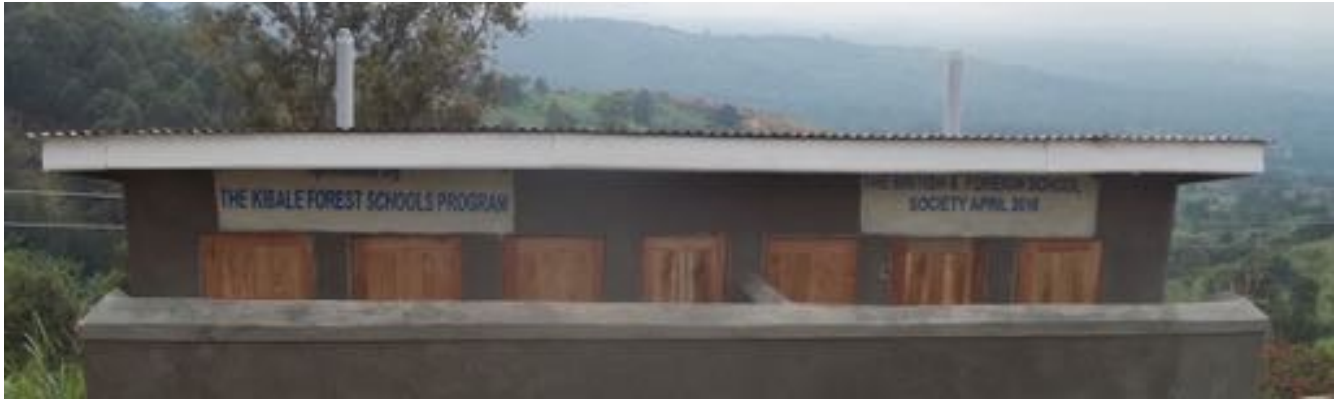
New Girls Latrines and Washrooms at Iruhuura Primary School
