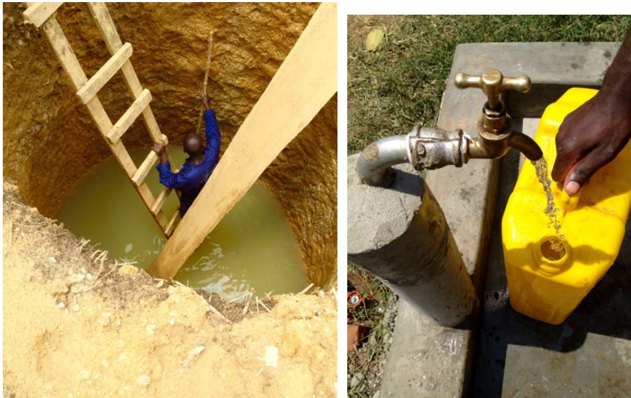
Digging Farm Well and the first water through the taps.
