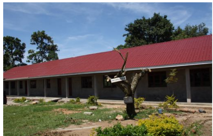
New Kigarama Classroom Block
