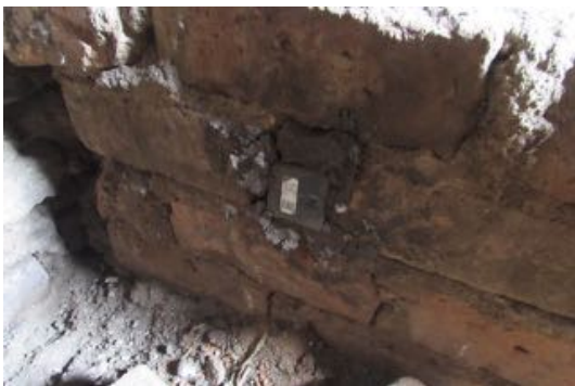
Stove use sensor in place
